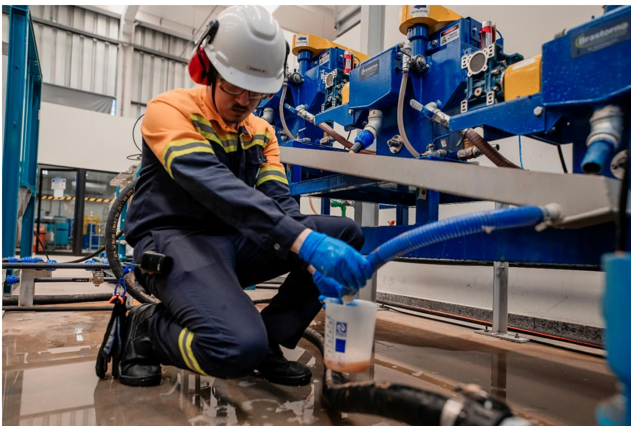
Figure 11: Process sample collection during commissioning.
