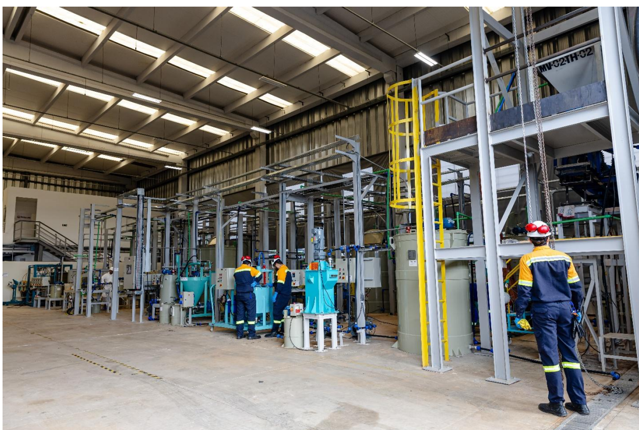
Figure 3: Stage 1 Beneficiation Facility Overview - 100 kg/h Capacity.
