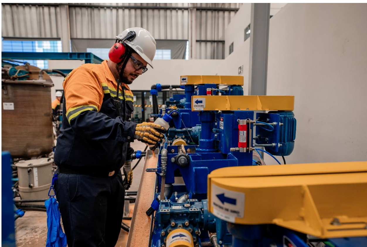
Figure 9: Flotation solution dosing during commissioning.
