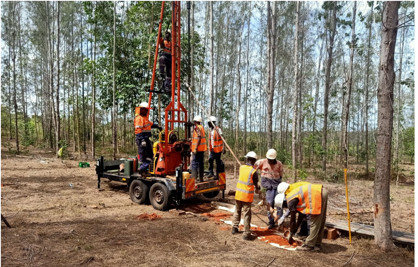
Figure: Auger drill rig in Kwale East.
