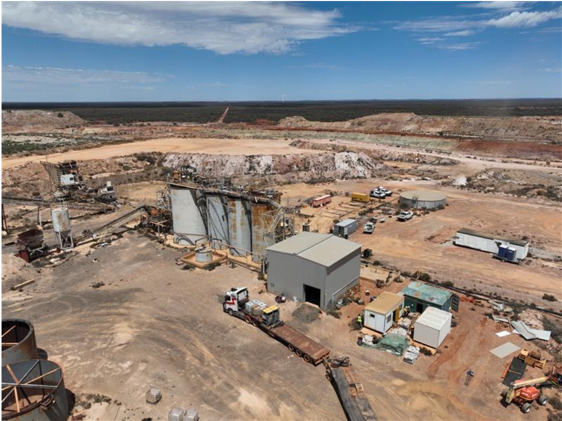
Figure 1 - Brightstar legacy processing plant site (Dec '25)
