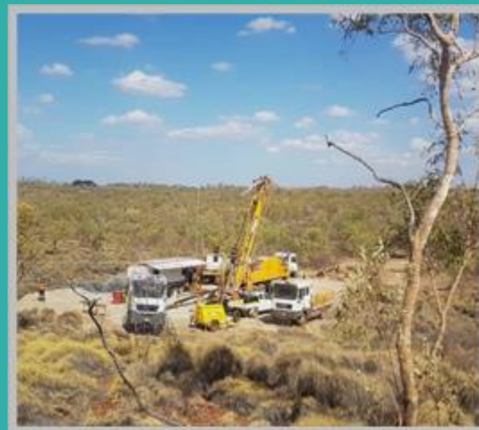
Drilling underway, Mackenzie Springs, October, 2020
