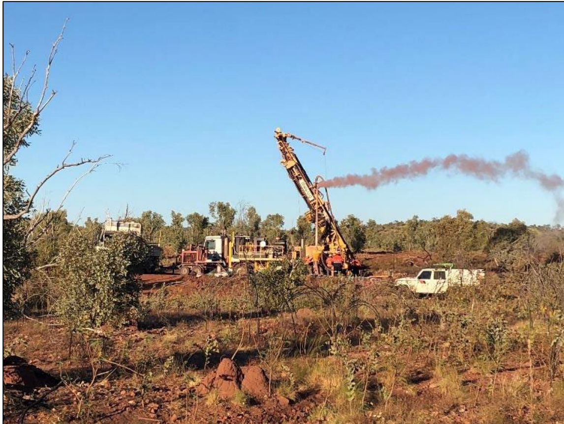
FIGURE C-4: DRILLING OF BO_332RC
