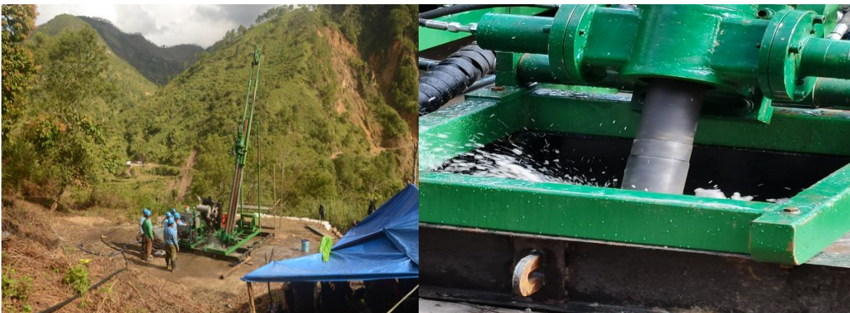
Image 1. Drill Rig at MCB 33 in operation
