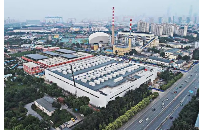
Worlds largest Vanadium battery Dalian Province China, 100MW/ 400MWh and enough power to meet demand from 200,000 residents
