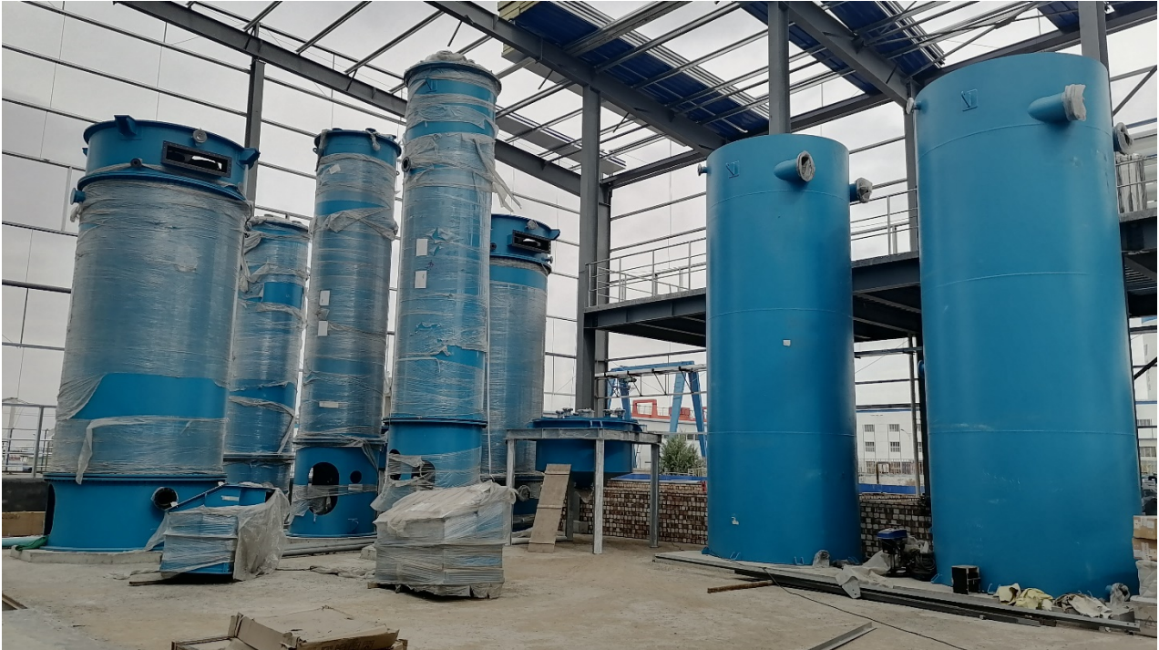
Photo of the CIF® columns and bioreactors being installed on site at Ordos
