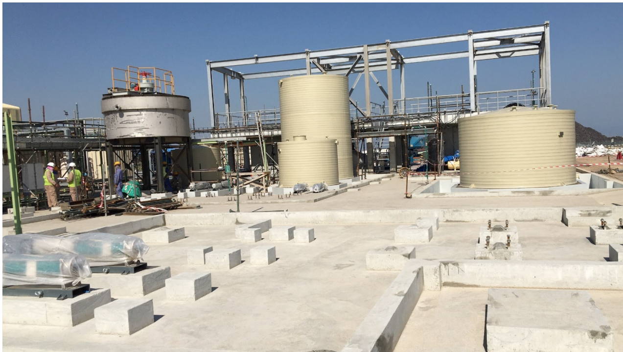
Photo of the installed clarifier and footings for Clean TeQ Water's equipment in Oman
