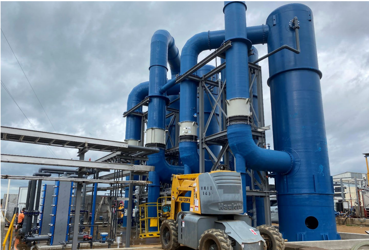
Installation progress of the EVAPX® system at the customer's site in New South Wales
