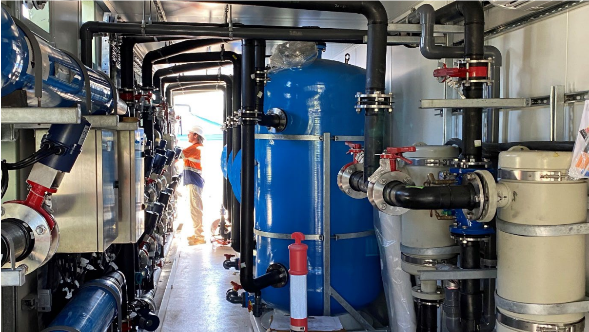
Inside view of the containerised Koumala bore water treatment plant
