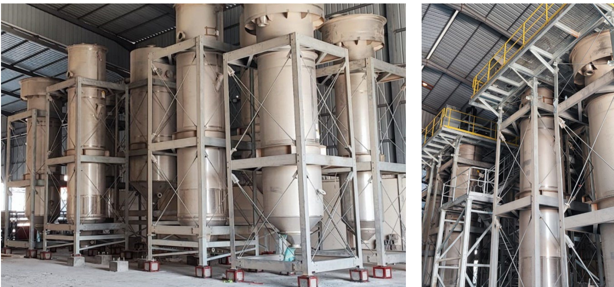
CIF® columns arriving on site and construction of upper platform
