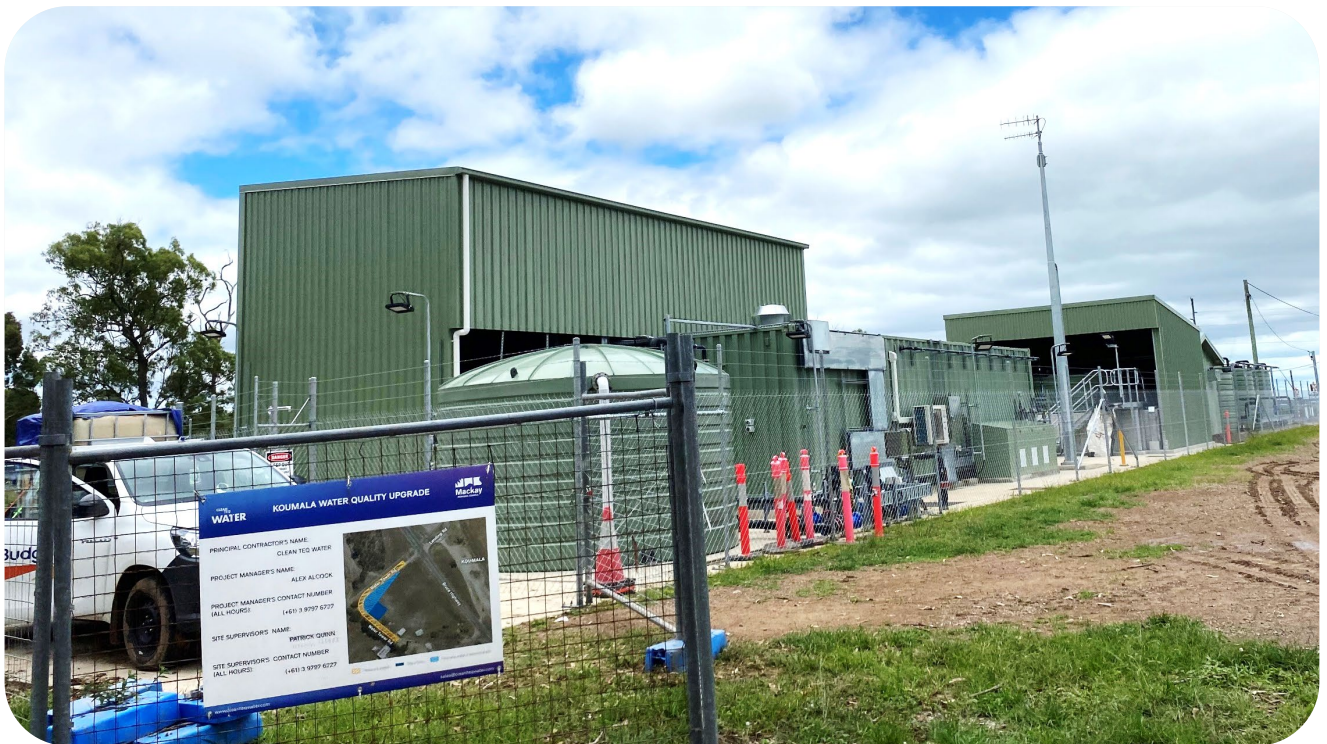
Photo of the Koumala water treatment plant site
