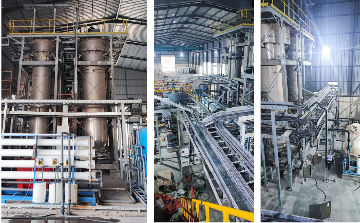
Installation progress of the NESR HIROX® plant
