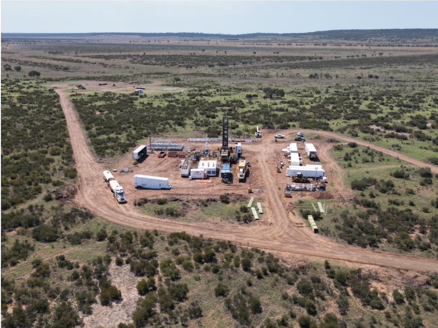
Figure 2: Aerial shot during drilling of ME2 (lateral well) looking northwest towards ME1 (vertical well)
