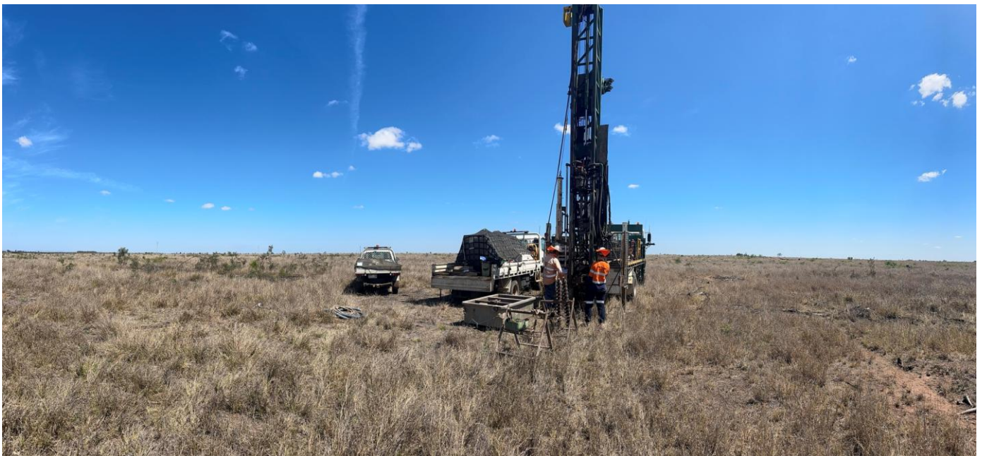
Figure 3: Geotechnical soil sampling along proposed pipeline route to confirm soil and rock technical parameters for design and construction work
