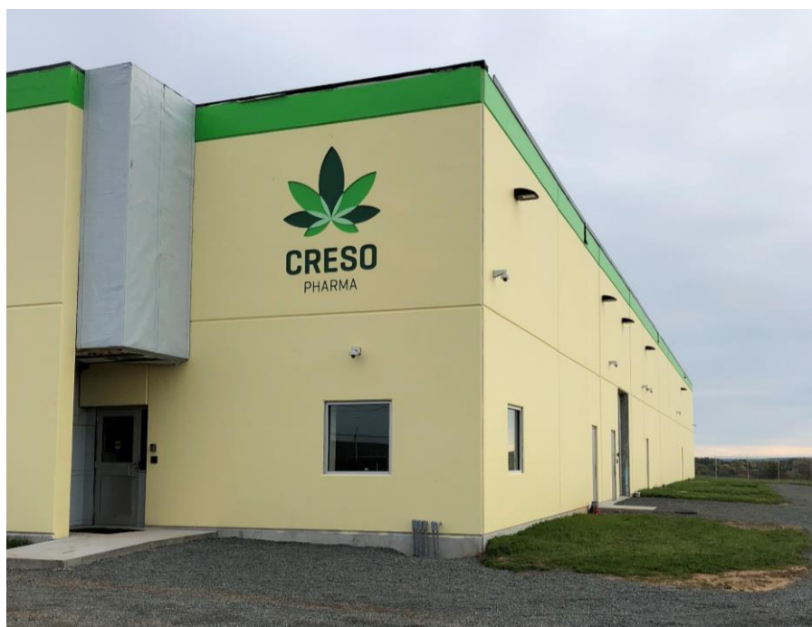
Figure 1: Mernova growing facility
