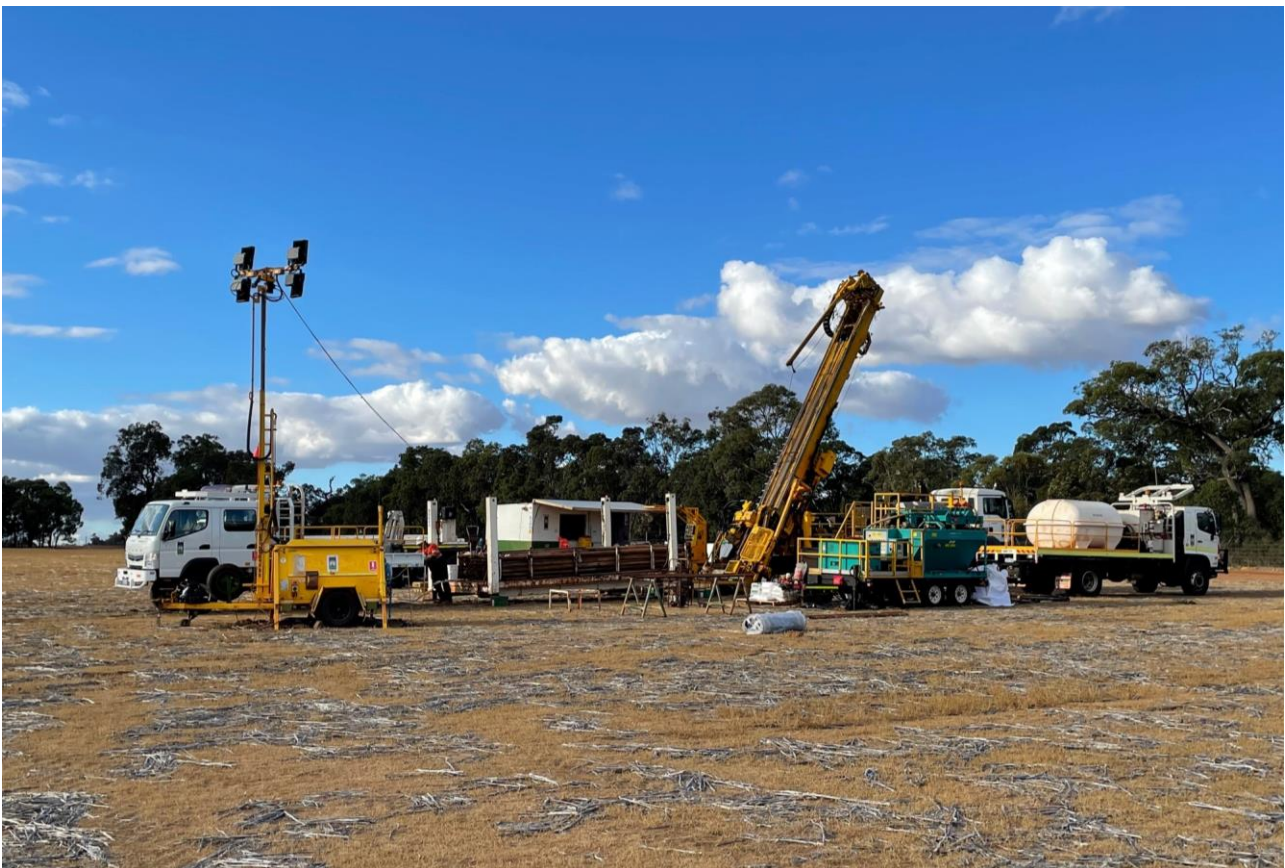
Figure 1. Drilling at XC-29, Yarawindah Brook Project.
