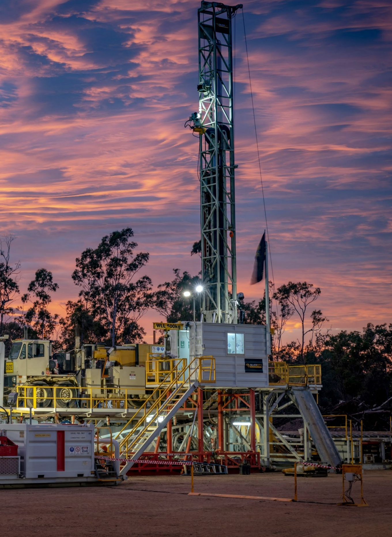
Drilling at Range-7 Photo by Alan Johnson
