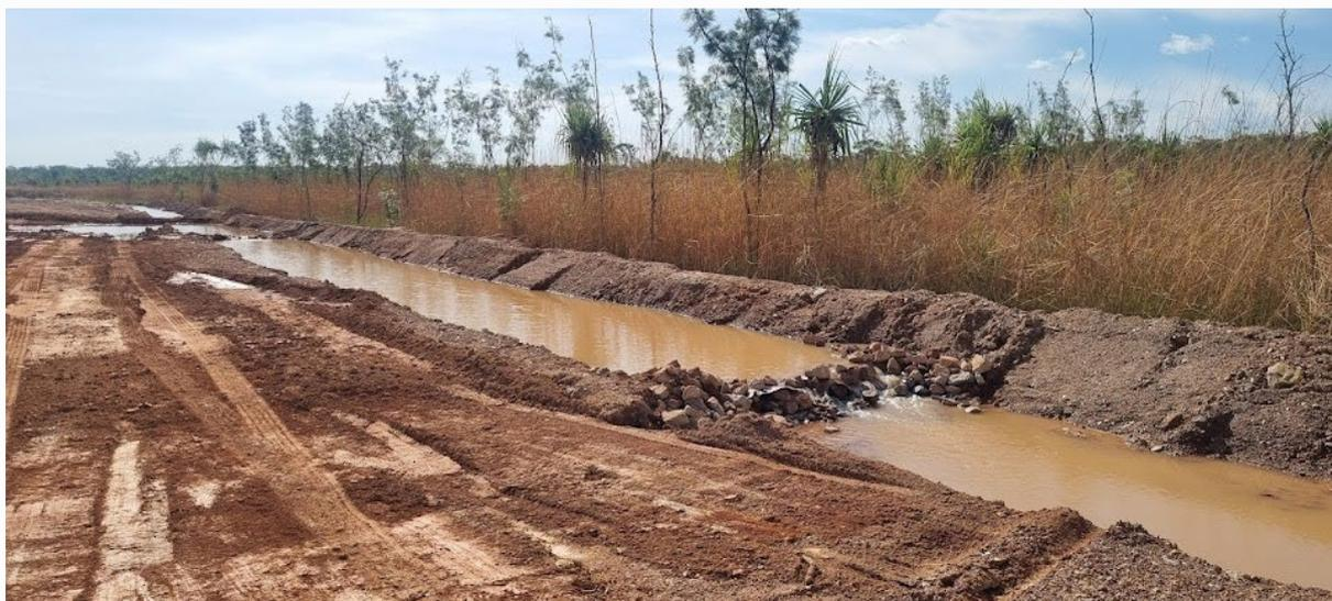
*Figure 6. Sediment Basin #2 (nth end) passive drainage*
