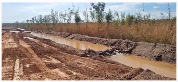
Figure 6. Sediment Basin #2 (nth end) passive drainage
