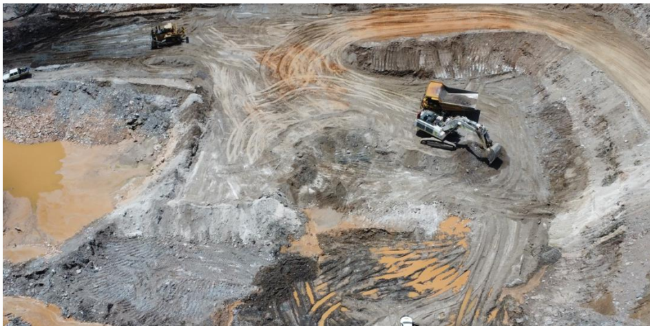
Dewatering of the Grants Pit was safely completed, and water management across Finniss is under control allowing for full mining operations to recommence in late March 2023.
