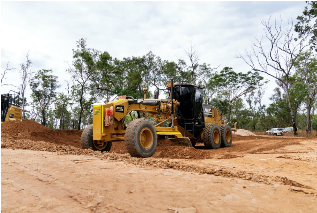
BP33 surface works underway
