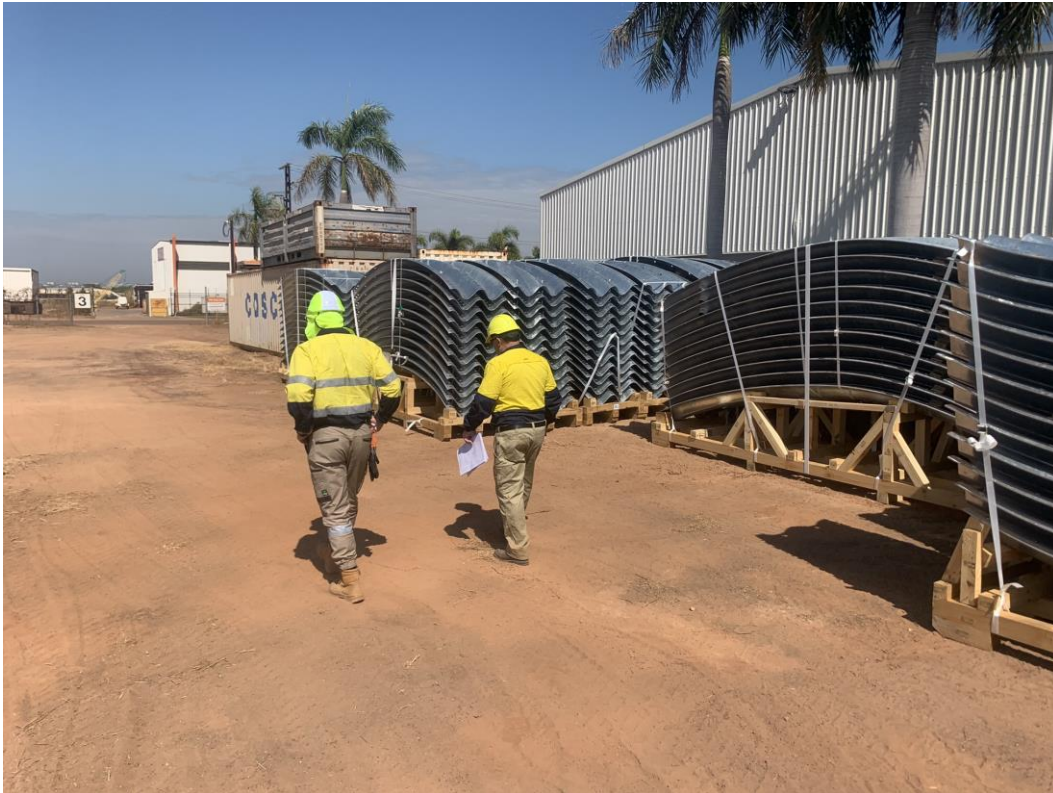
Tunnel liners delivered to Darwin laydown area
