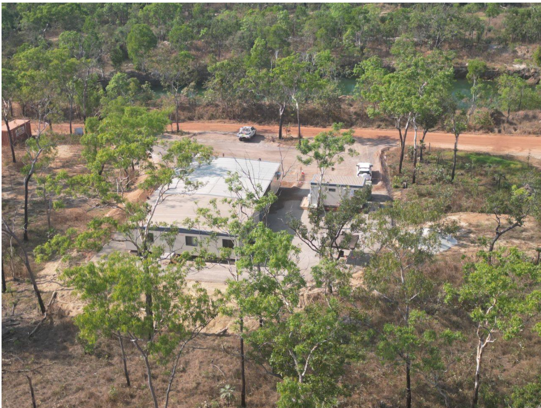
BP33 site buildings established
