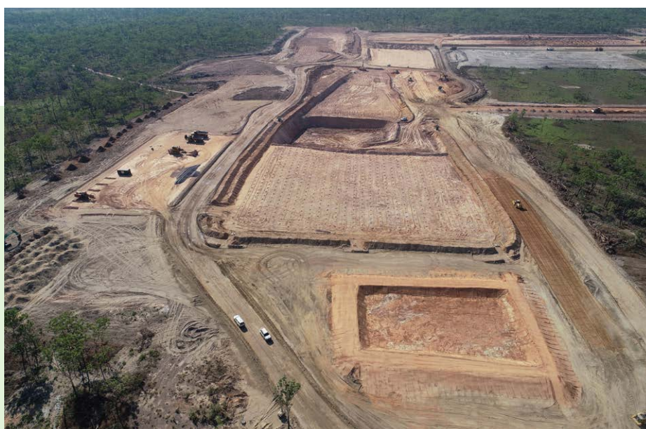
BP33 aerial view early September 2023. Box-cut excavation commences.
