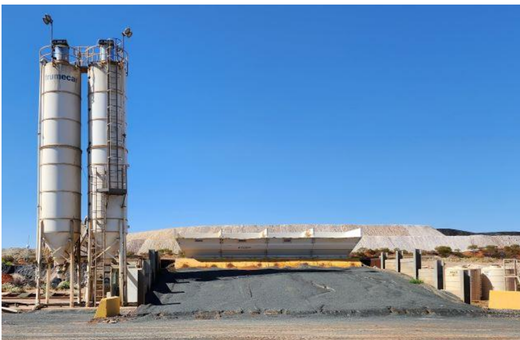
Image 10 / Concrete batching plant cleaned and serviced – ready to go
