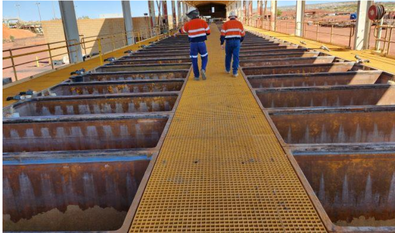
Image 6 / EW cells stripped of anodes and cathodes, cleaned and hydrottested waiting for refurbishment
