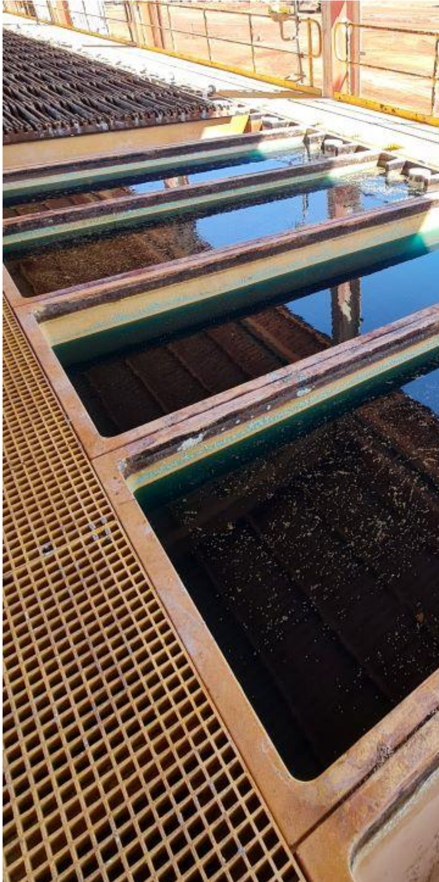
Image 5 / Hydro testing EW cells following removal of cathodes and anodes and clean up
