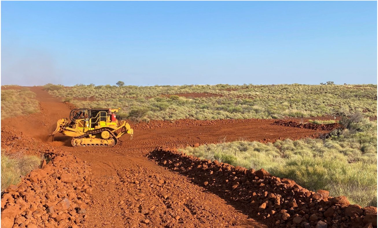
Photo 1. Drill pad clearing for diamond drilling (DSO iron ore on surface)
