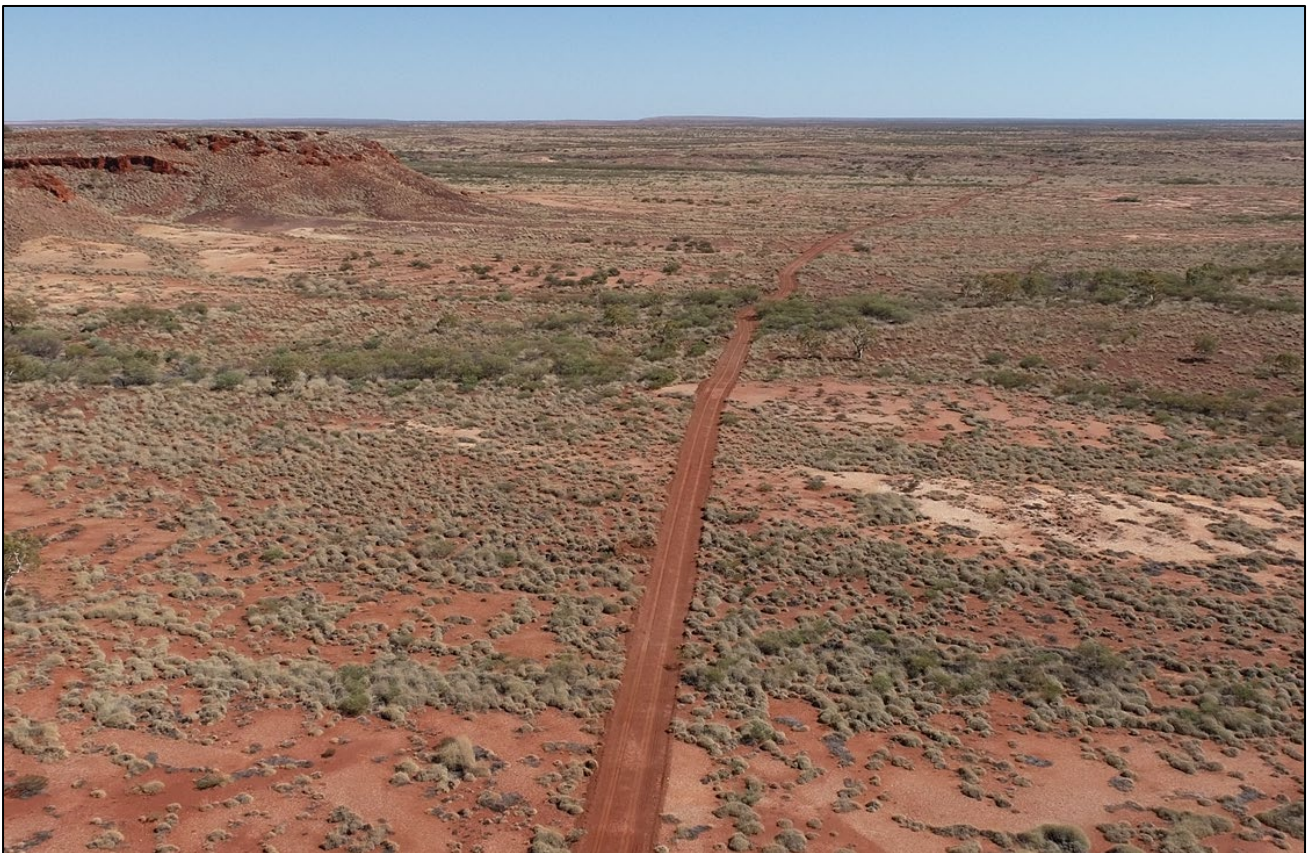
Figure 3. Access track constructed along the proposed haul road corridor, linking Robe Mesa to the Northwest Coastal Highway
