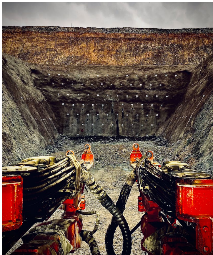
Dev Mining Services at the Mt Marion Site
