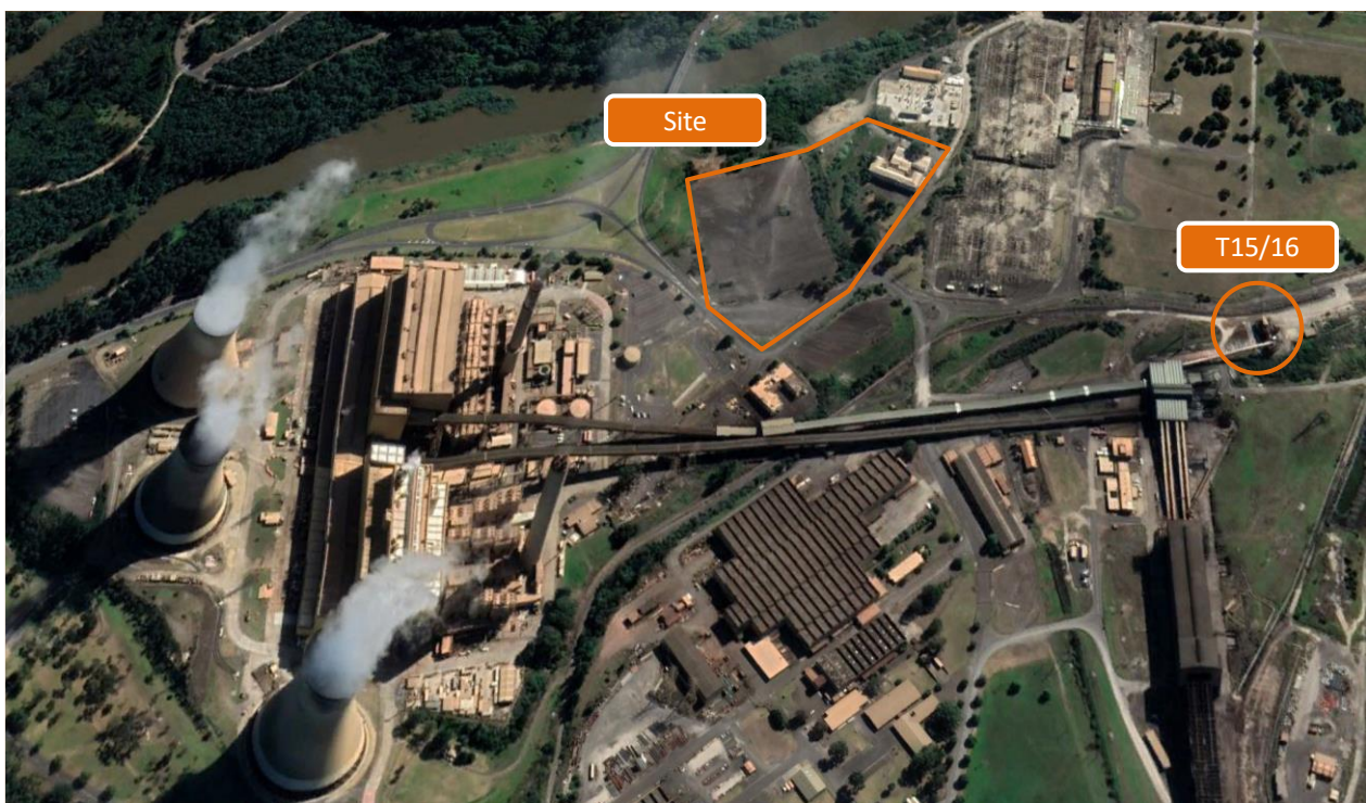
Above: Overview of the Yallourn power station, with the recently purchased property highlighted (site) in proximity to the current lignite terminal upgrade (T15/16).
