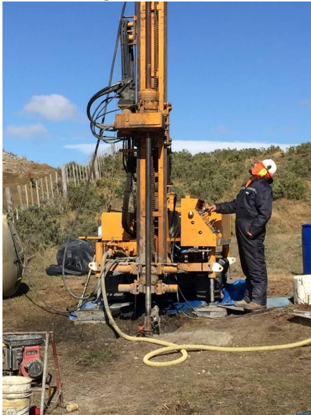
Photo 1. Drilling Commences at Mina Rica
