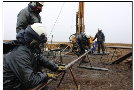
Photo 3. Extracting core
