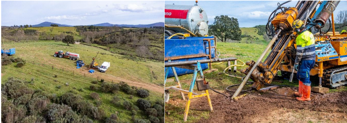
Aerial view and detail image of drilling rig.
