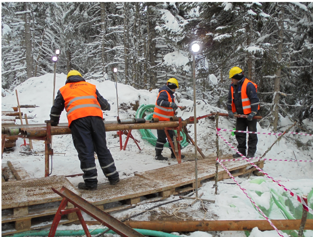
Figure 1: Disconnecting the pulled rod for drill core retrieval.
