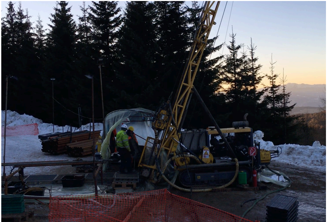
Picture 1: Drill rig positioned
