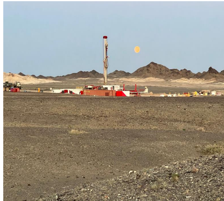
Pilot well drilling at Nomgon
