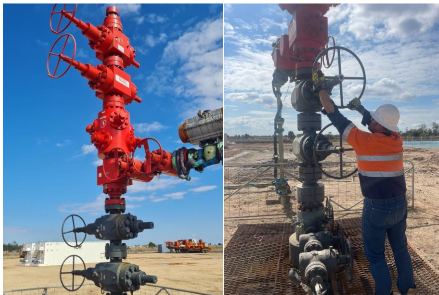
Servicing of well head at Daydream-2
