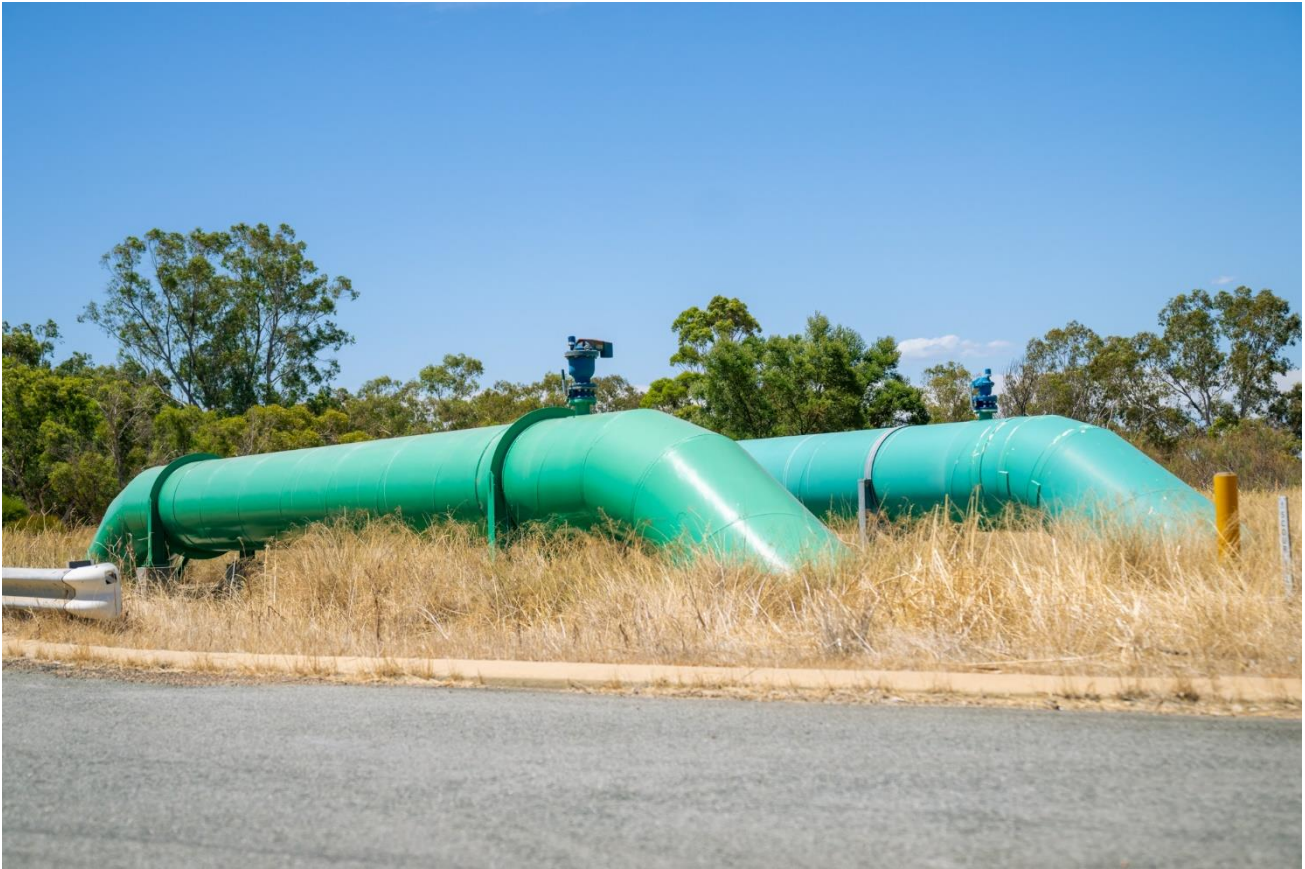
Image 2: Stirling Trunk Main pipeline outcropping at the Project
