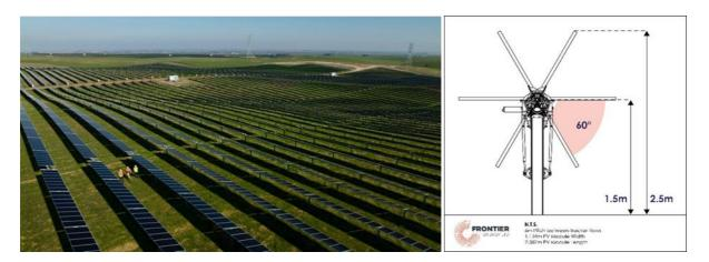
Figure 11: Typical solar farm arrangement with tracker
