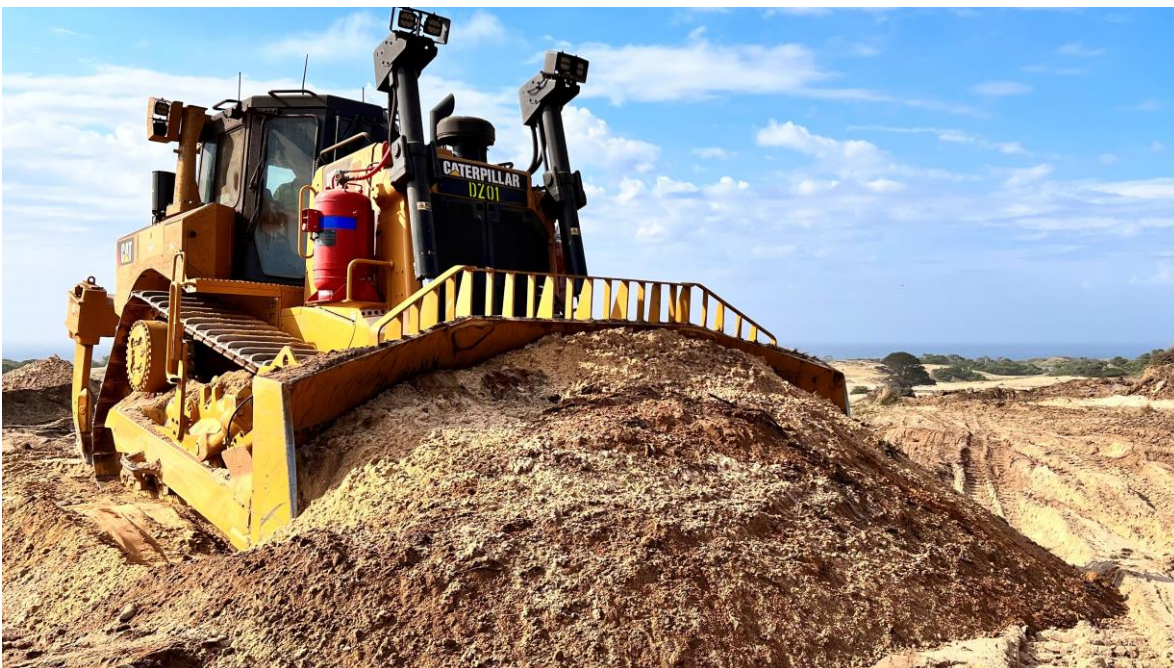
Figure 1. Construction commences on site at the Dolphin Tungsten Mine
