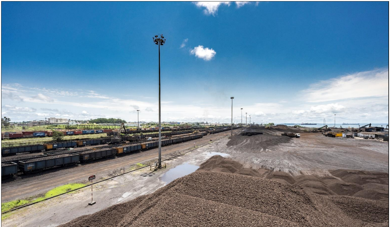
Figure 2: Rail and port facilities at the Owendo Mineral Port
