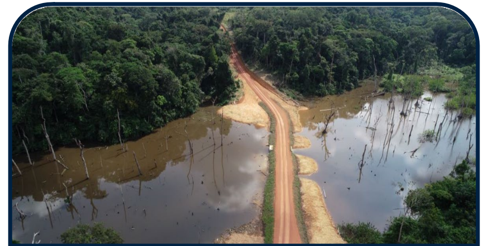
Resurfaced Tsengué Base Camp access road.
