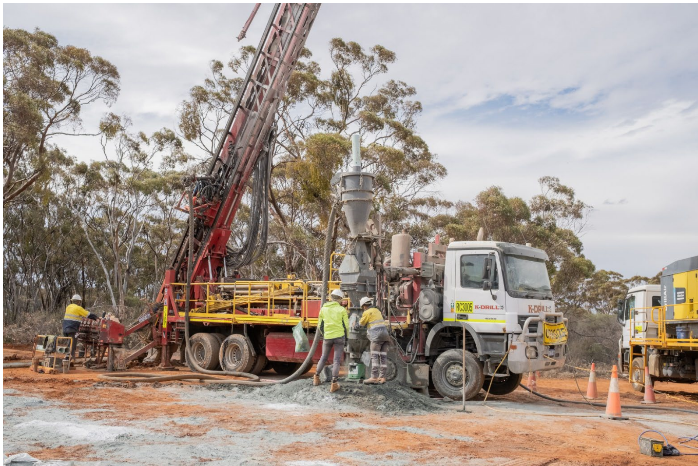
Figure 6. K-Drill RC drilling rig setup at the Manna Lithium Project.
