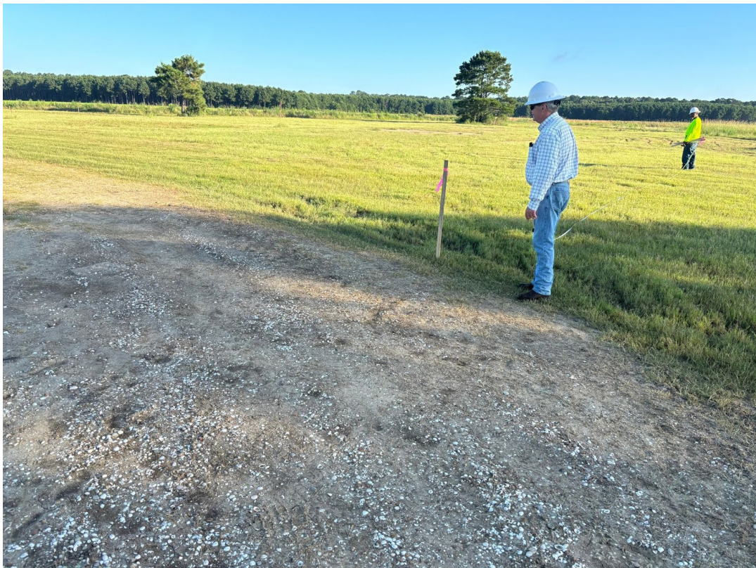
Figure 1: Site preparation activities at Zydeco-1
