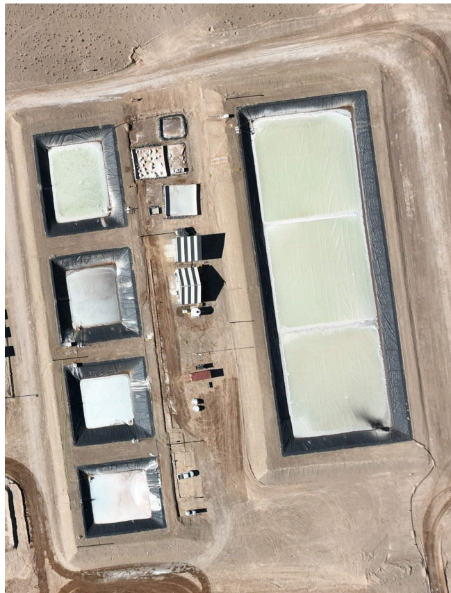
Figure 4: Aerial view of existing pilot plant
