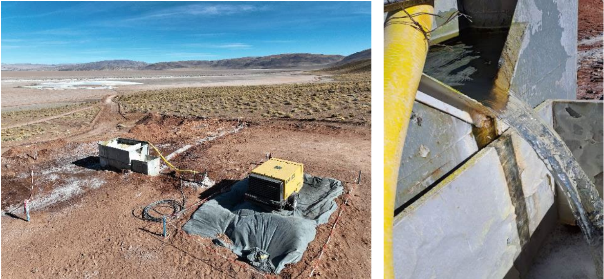
Figure 6: View of C-02-23 exploration well and ongoing airlift test.
