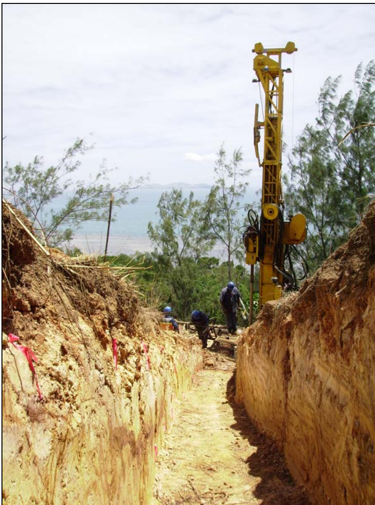
Figure 5. Northern end of trench FT1 at the NE Gossan zone of the Faddy's Gold Deposit. Note that the mineralized gossan is mostly soft, poorly indurated rock and that soil cover is thin.
