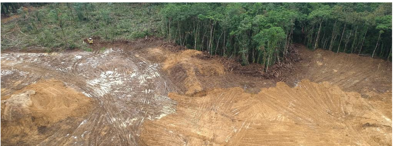
Figure 4: Plant Site Clearing
