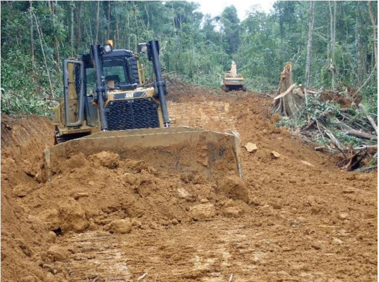
Figure 5: Wharf road pioneering works
