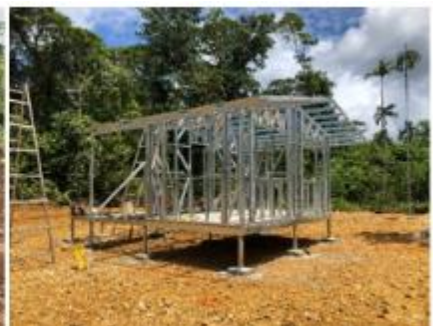
Figure 8: First houses erected
