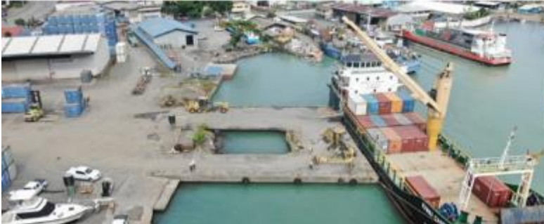
Figure 9: Barge departing from Lae
