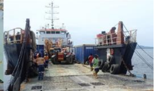
Figure 10: Barge arriving on site
