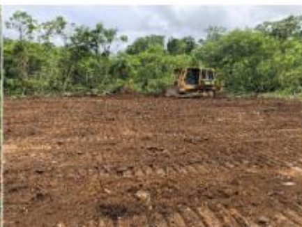
Figure 7: Village site preparation
