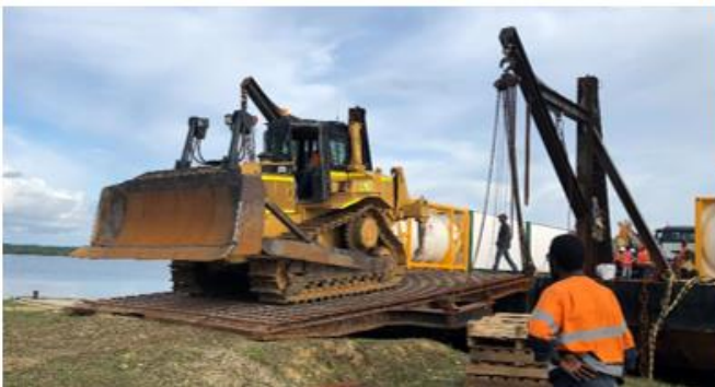
Figure 2: Equipment Mobilised to site by Barge
