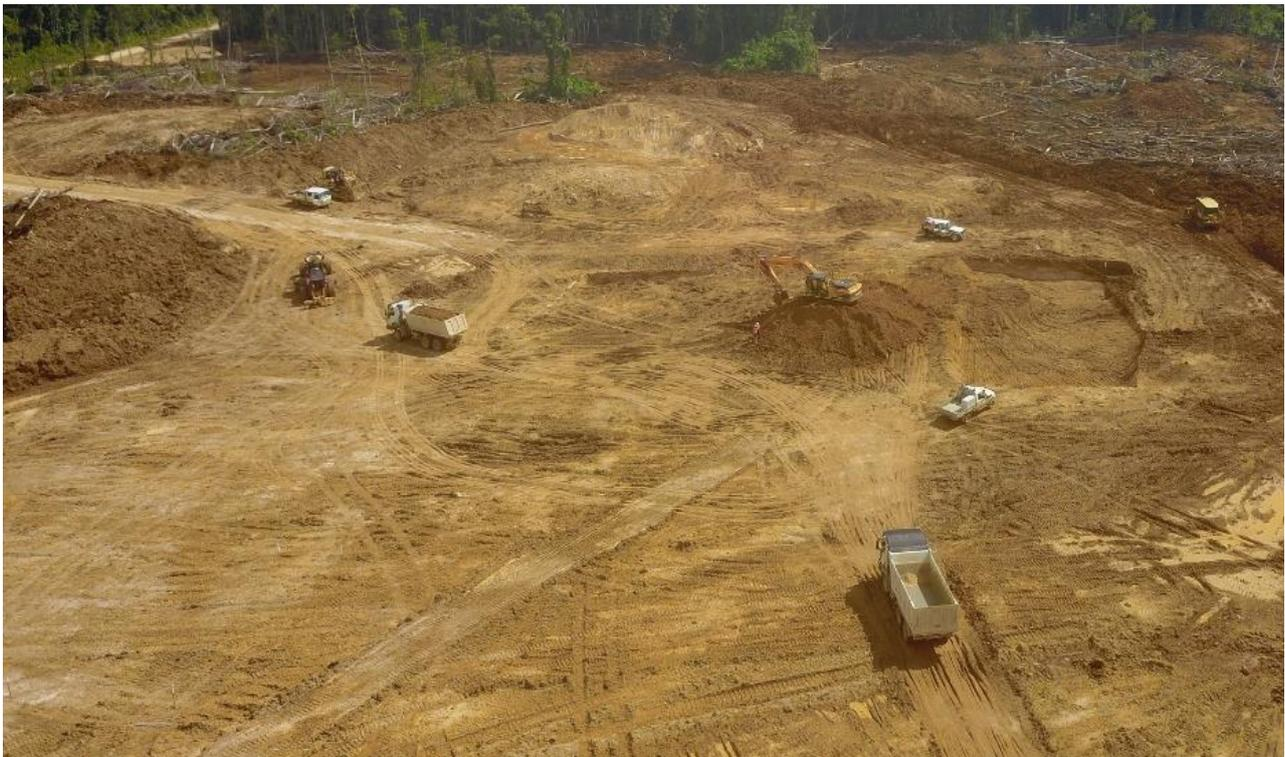
Figure 1: Commencement of processing plant infrastructure: box cut for CIL tanks
