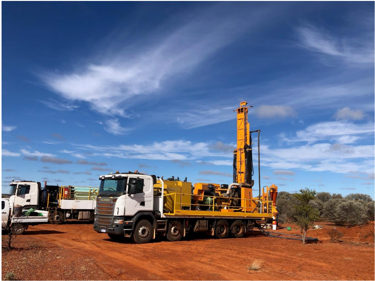
Figure 2. RC drill rig on site ready to drill at Copper Ridge
