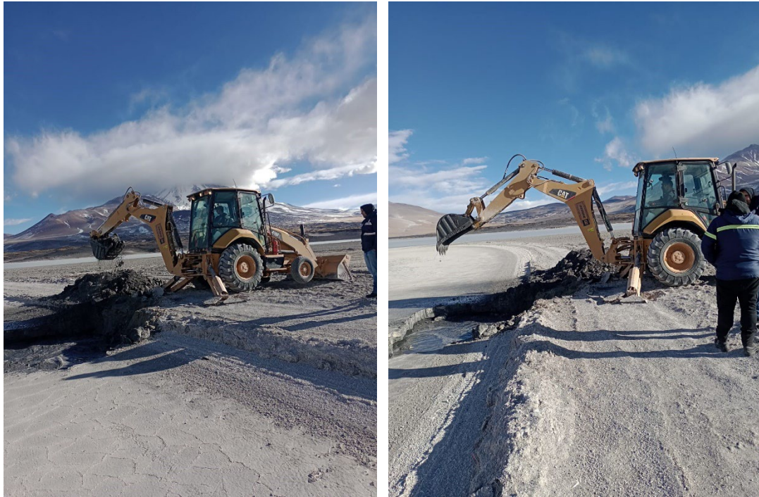
Figure 3 Preparing drilling fluid supply for SJDD01, San Jorge Project
