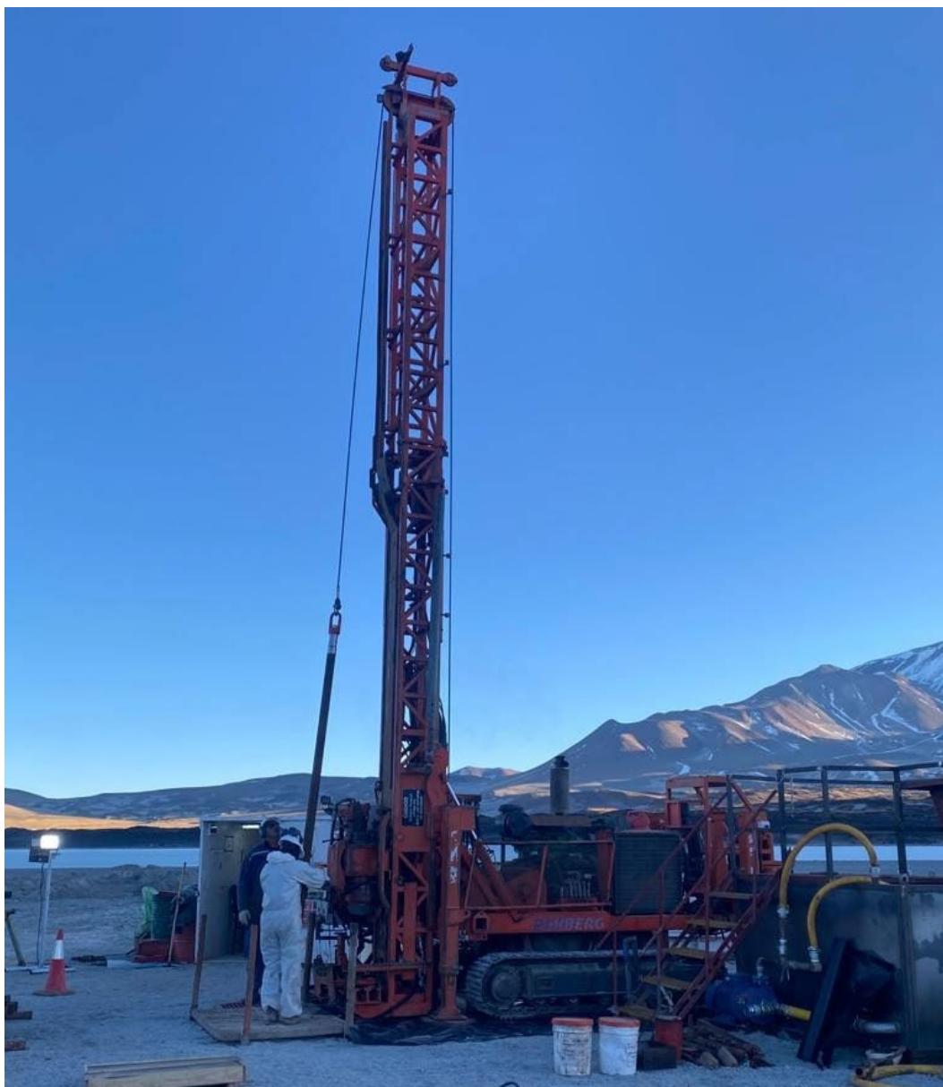
Drill rig commencing drilling at the San Jorge Lithium Brine Project.
