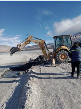
Figure 2 Preparing drilling fluid supply for SJDD01, San Jorge Project
