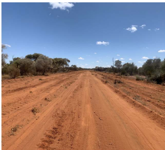
Figure 1: Northern Haulage Road Clearing
