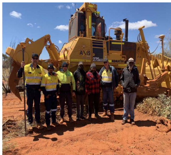
Figure 2: PRG workers, Martu Monitors and Earthmoving machinery. Commencement of Development Operations
