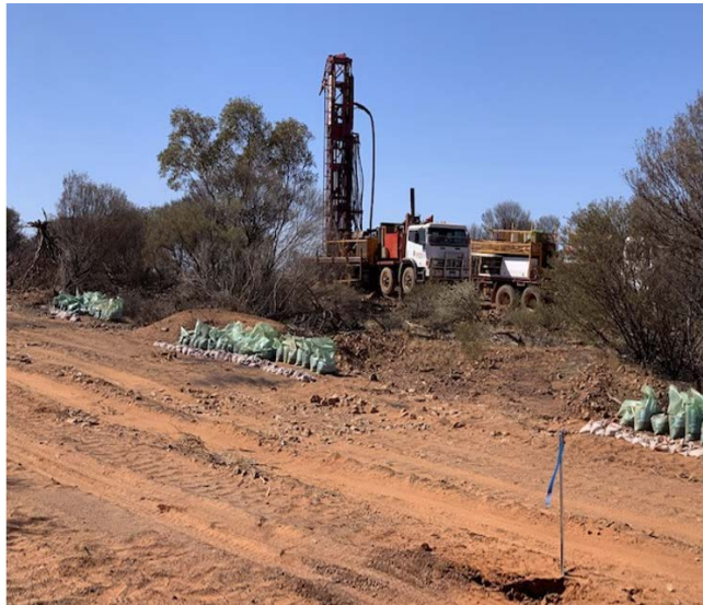
Figure 3 - RC drill rig at Wiluna West completing grade control drilling
