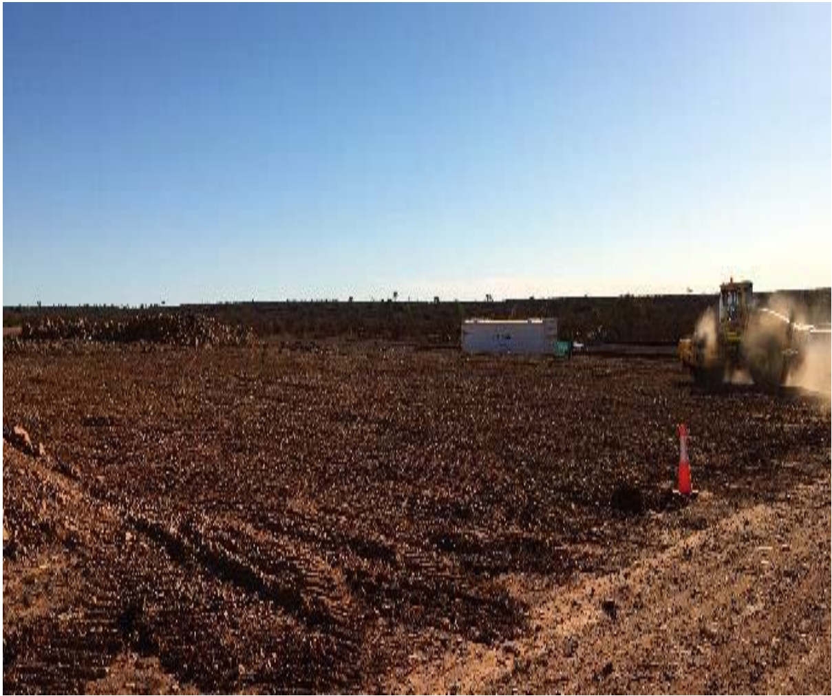
Figure 4 – Drill & Blast Laydown Area
