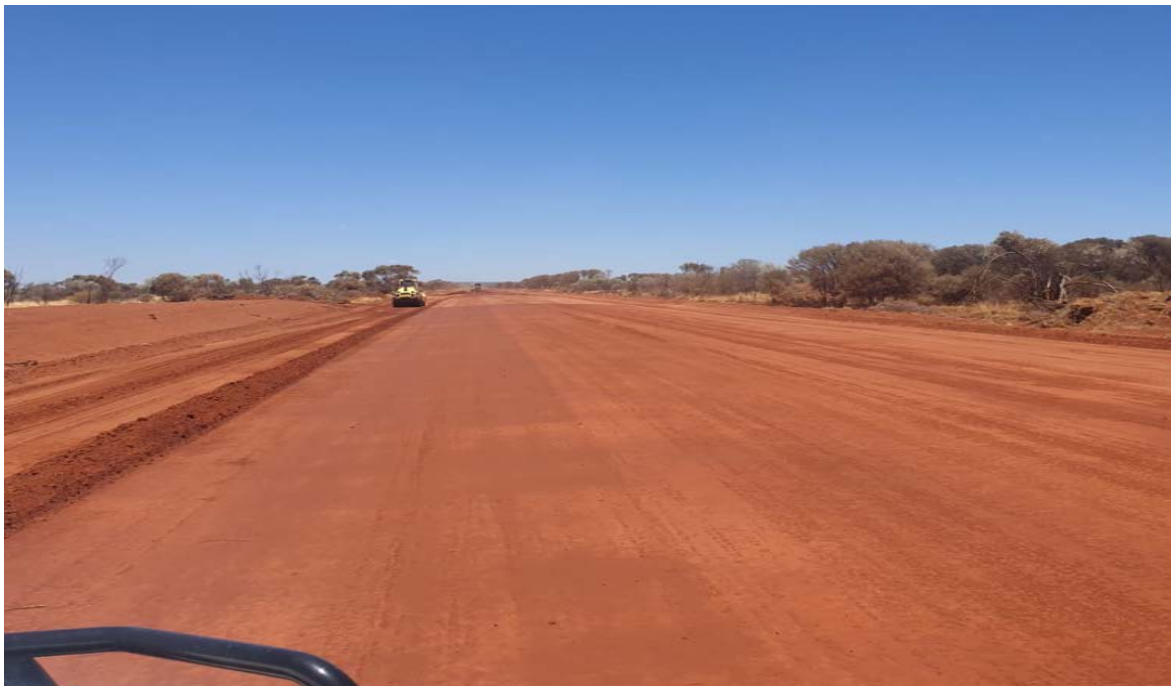
Figure 8 – The Northern Haulage Road under construction
