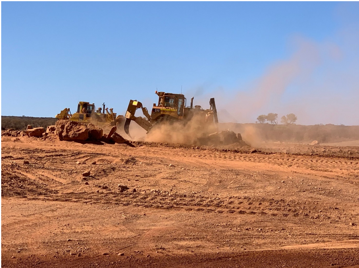
Figure 5 – Crusher Pad Earthworks
