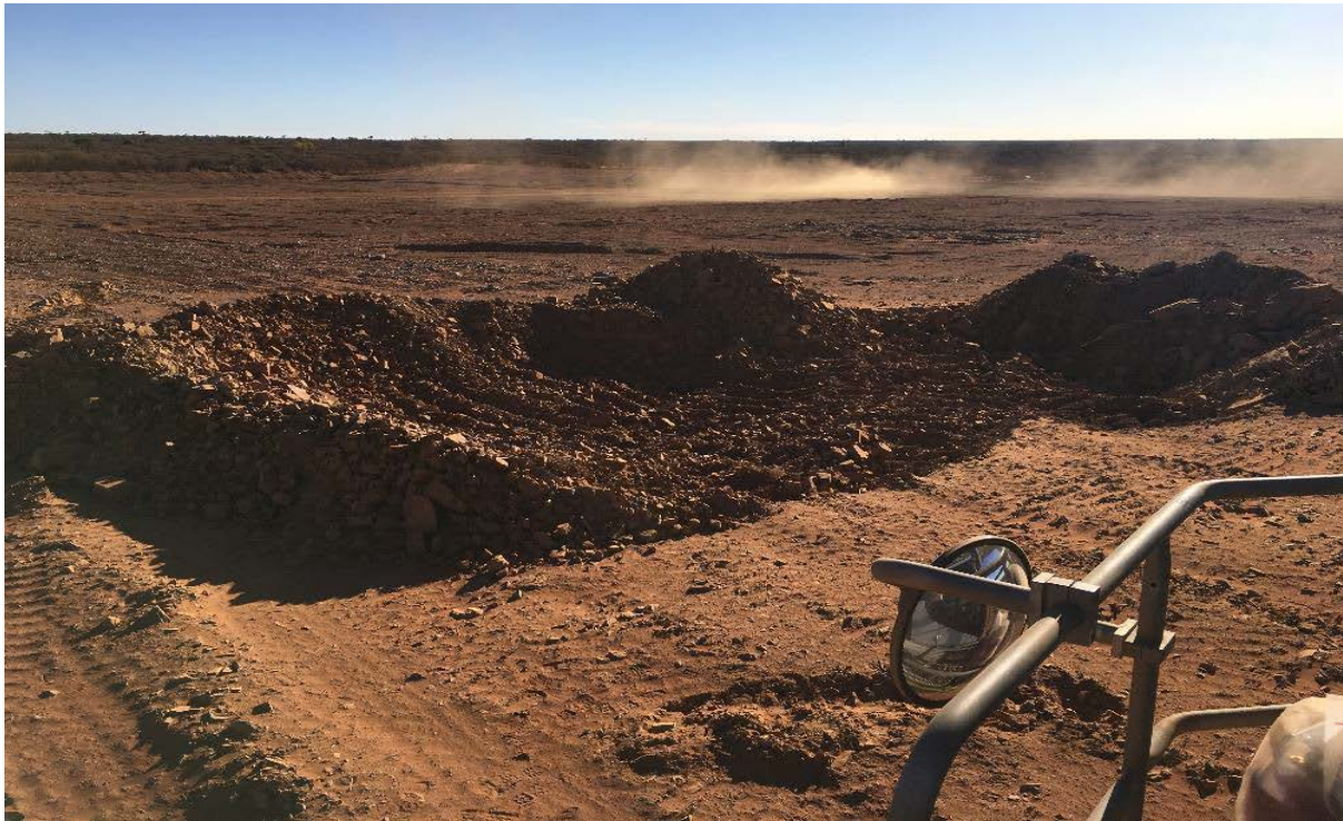
Figure 2 – Start of Cut and Fill for the ROM Pad.
